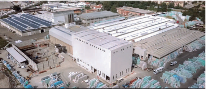
SASSUOLO TILES (Atomizer and Warehouse)
